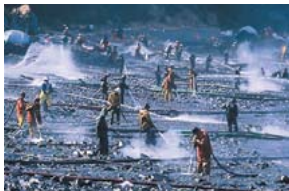
Exxon Valdez oil spill workers use pressure washers to wash oil from the beach on Smith Island, Prince William Sound. The oil was impounded in the water off of the beach and skimmed from the water. May 2, 1989.
